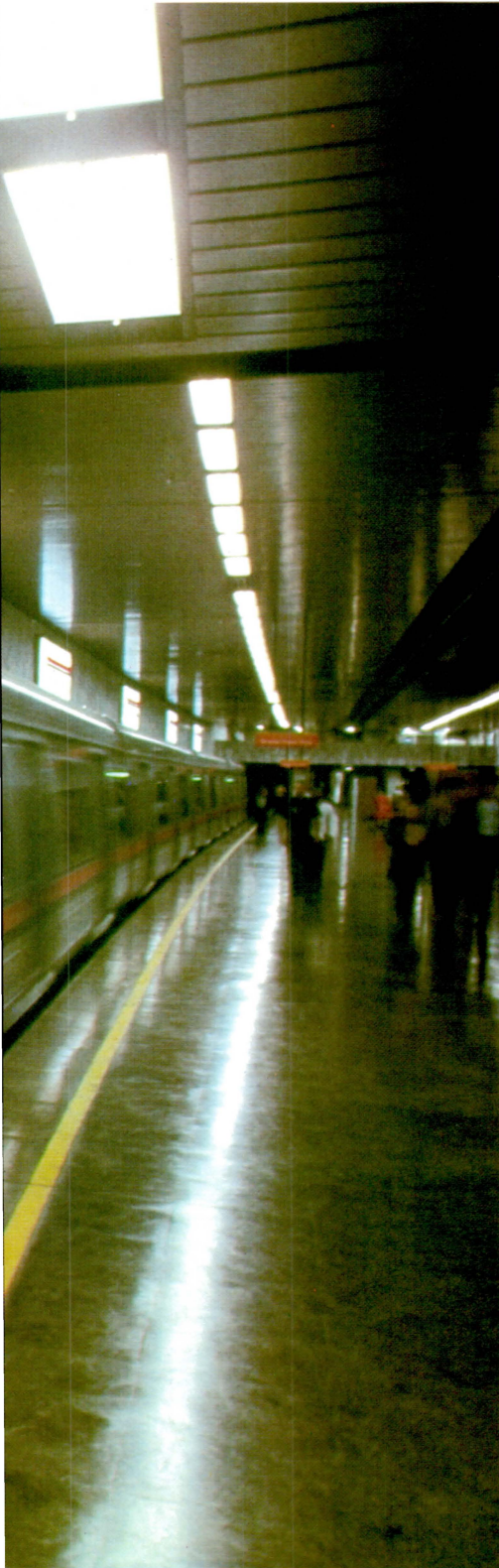
Brazil's new Metro subway system, nearing completion in Rio de Janeiro, has trains departing every 90 seconds and more than 80,000 riders per hour using the system — all being monitored by eight PDP-11/70 computers in a central control room. When completed, the 20-mile Metro system will be one of the most sophisticated public transportation networks in the world.
